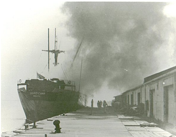
FIG. 18. Looking east along north side of Warehouse '90' showing the S. S. GRANDCAMP a few minutes before the explosion.
