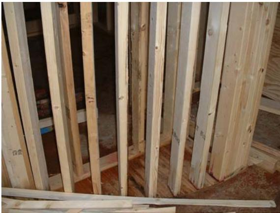
Don't try to breach a curved wall framed with either steel or wood studs. Curved walls have studs spaced more closely than the 16-inch, 18-inch, or 24-inch centers that are common in straight walls to provide support for the multiple layers of drywall board that will be used. Photo 1 shows a curved wall framed with wood studs on six-inch centers that will be covered with at least two layers of ¼-inch drywall board, which is more flexible and can
