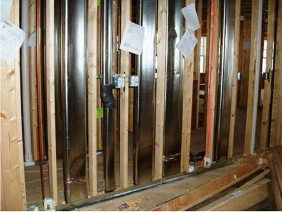
Breaching a straight wall may not create a usable opening. Photo 2 shows a wood-frame wall in a new home, with studs on 16-inch centers. Only two of the stud spaces shown might be usable for entry or exit openings. The rest contain electric cables and boxes, steel dryer vent pipe, steel ducts, steel gas pipe, and plastic drain-waste-vent pipe. Unless we are very familiar with the building, we won't know this until we have spent
