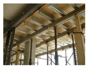
Photo 3 shows the completed forms and supports for the extension of a second-floor terrace at a restaurant. The formboards are oil-treated plywood on crisscrossed extruded aluminum alloy beams, supported by adjustable columns and bracing of both steel and wood.
