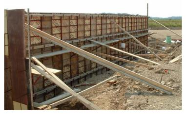
Photo 1 shows the nearly-completed forms and supports for a 16-inch-thick load-bearing wall for a factory. From footing to top of the form, this wall is 16 feet high. The concrete form panels are plywood set in steel frames that are pinned to the top of the concrete footing and connected to each other by "wedge-bolts." The panels are
