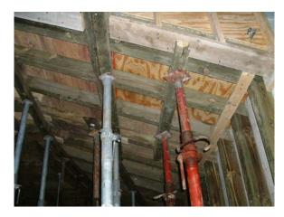
Photo 2 shows part of the completed forms and supports for the floor in an auditorium, with a sloped reinforced concrete floor and rows of seats on concrete steps that will be poured as part of the floor deck. The formboards are oil-treated plywood on wood beams, supported by adjustable steel columns. This is a variation on the traditional falsework which included wood formboards, beams, columns, and bracing.
