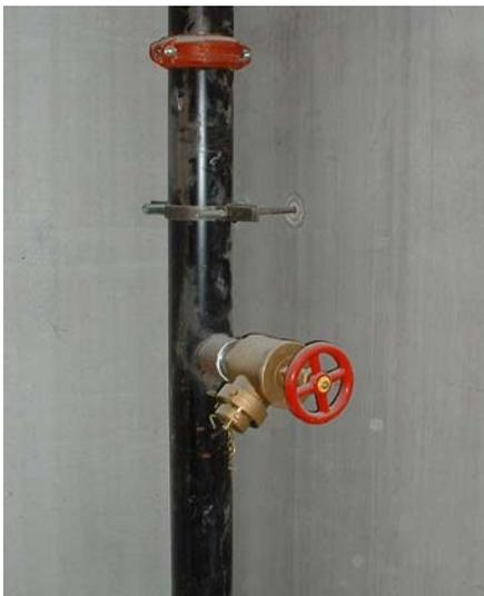
Class I and Class III standpipes may have fire department connections to supplement the building water supply.
