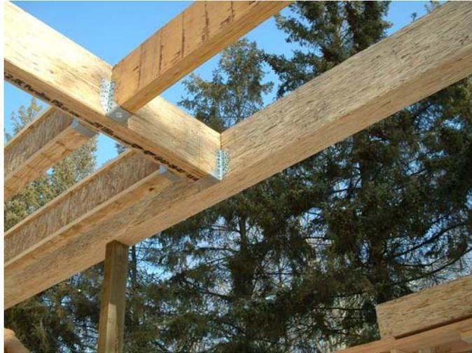
One manufacturer will allow holes to be cut horizontally through PSL girders and beams only if they are in the center 1/3 of the vertical dimension and only in the center 1/3 of the span. Only round holes are allowed. If there are multiple holes, they must be spaced so that there is at least twice the diameter of the largest hole between them. Square or rectangular holes or edge notches are not allowed.
