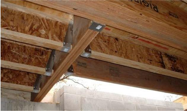
Photo 3 shows wood I-beams with LVL flanges and high-density oriented strand board (OSB) webs, supported by galvanized steel joist hangers from LVL beams and girders.
