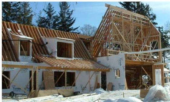
lumberyards in longer lengths than any sawn lumber, and are available by special order in almost any length. Photo 2 (above) shows a large house under construction. The rafters shown in the higher part of the house at the right are 40-foot 2 × 12 LVLs, with a 2 × 18 LVL ridge board. The rafters shown in the lower part at the left are 26-foot 2 × 10 LVLs with a 2 × 12 LVL ridge-board. Both roofs will be sheathed with plywood and covered with slate.
