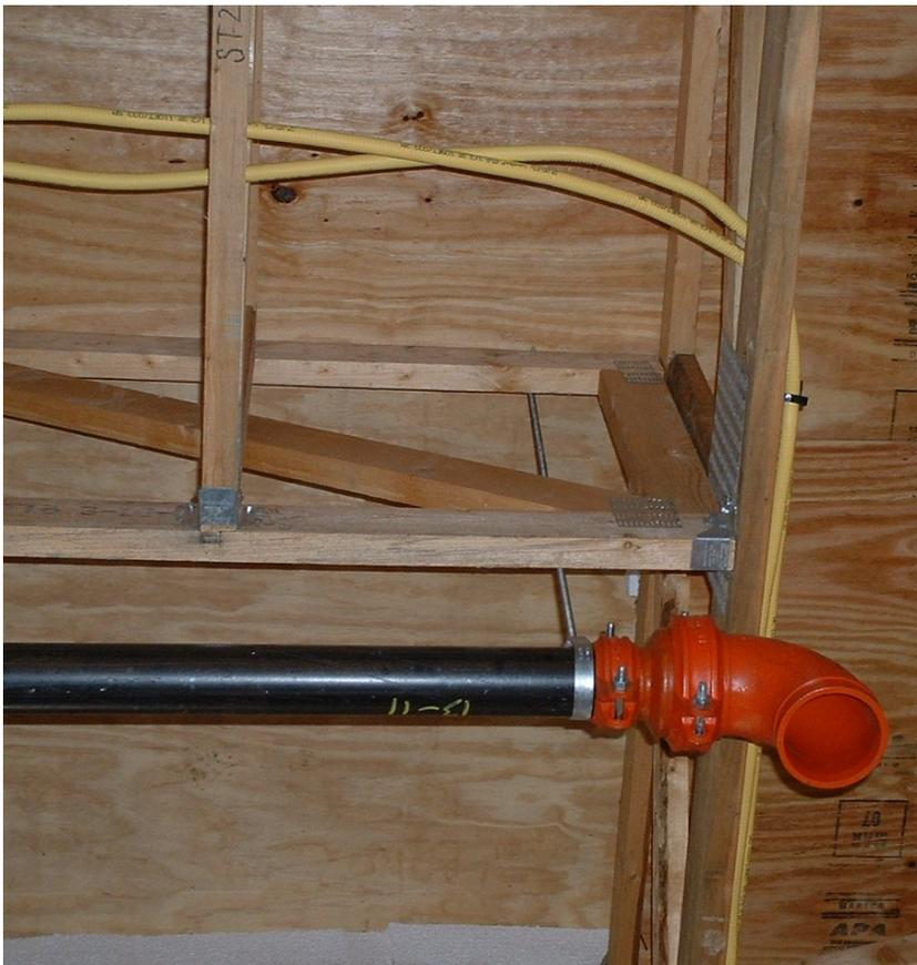
Photo1 shows a pair of plastic gas pipes supported by wood roof trusses in a strip mall under construction. Each will supply a water heater and heating unit for one of the mall's occupants. The large black steel pipe is the automatic fire sprinkler main, and the Victaulic elbow will be connected to the sprinkler riser.
