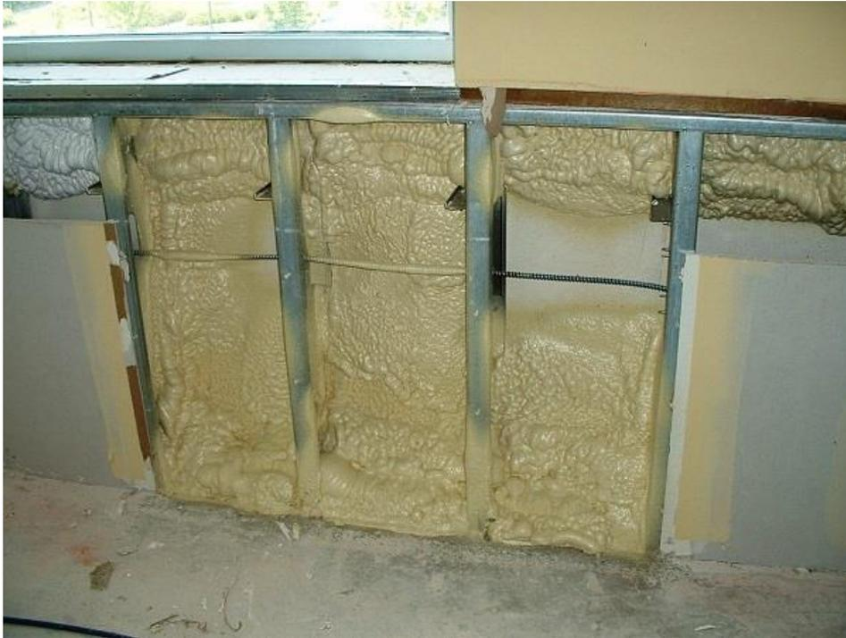
Photo 4 shows polyurethane foam that has been applied as insulation and vapor barrier inside a wood stud exterior wall.
