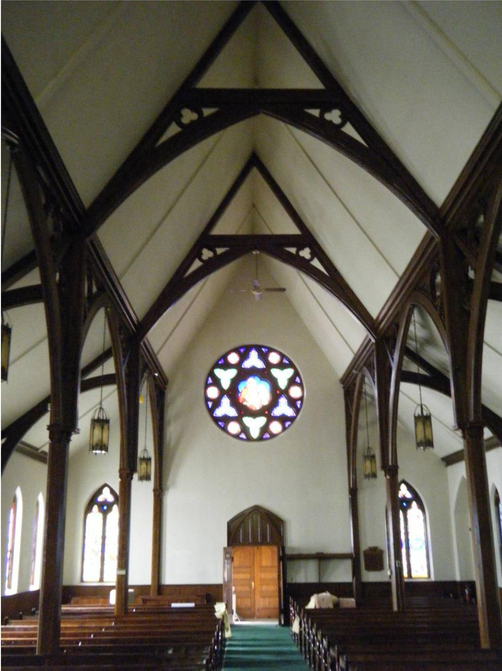
Photo 3 shows the trusses supporting the ceiling and roof assembly of a church, built in the late 1800s. The ceiling in this church is attached to the bottom of the same rafters that support the roof. These trusses are not only decorative—they support the ceiling and roof.
