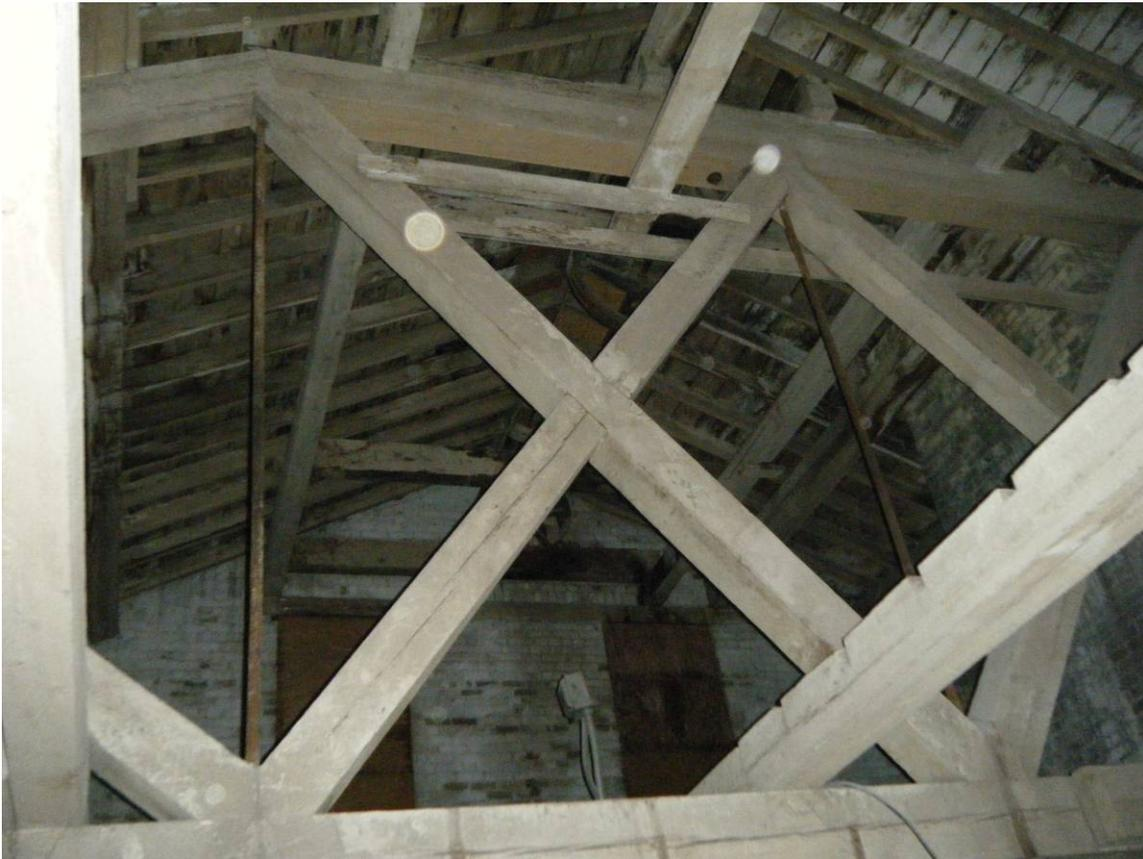
Trusses have been in common use in North America since before 1800. Some truss designs were developed for bridges and adapted for use in buildings. Photo 2 shows a timber roof truss in a “mill” (the ancestor of modern Type IV or heavy timber) building from 1840. The compression members of this truss are of wood, ranging from 8 x 8 inches to 12 x 12 inches (20.3 x 20.3 cm to 30.5 x 30.5 cm). The tension members of
